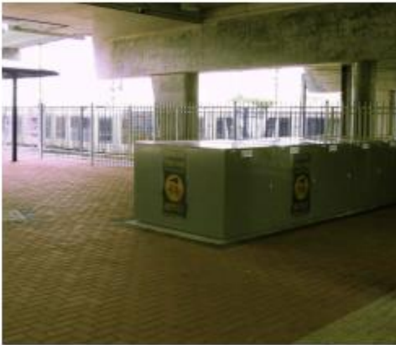
Photo 11.1: Bicycle locker installation at Liverpool Railway Station.
